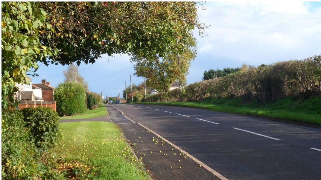
View into Deppers Bridge
